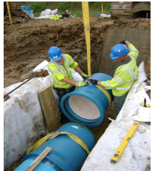
Plan and construction of new culvert from North Marsh into RSPB reserve.
