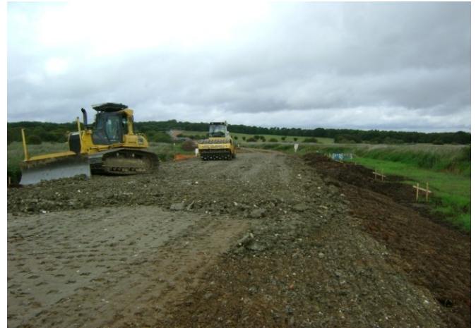
Placing and compacting clay layers
