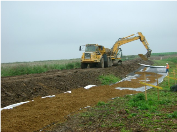
Placing geotextile and granular foundation
