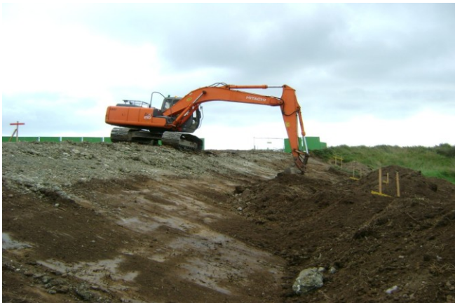
Cutting to surface of clay at an angle of 1 in 3
