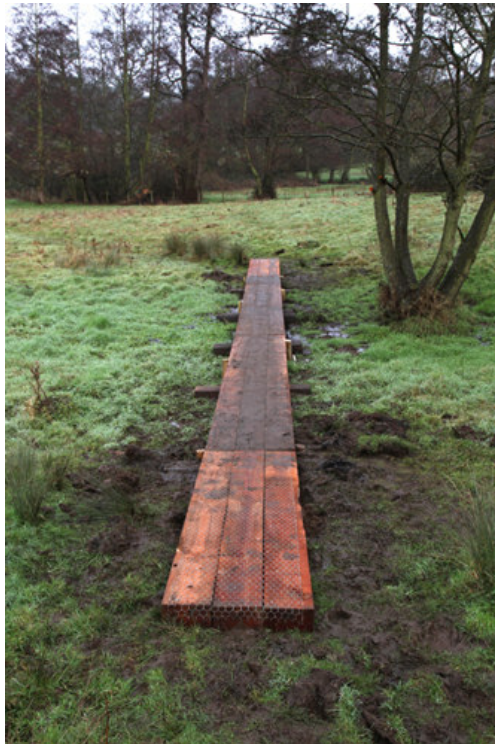
new sleeper walkway
