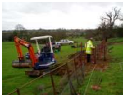
Kevin King installing new fence
